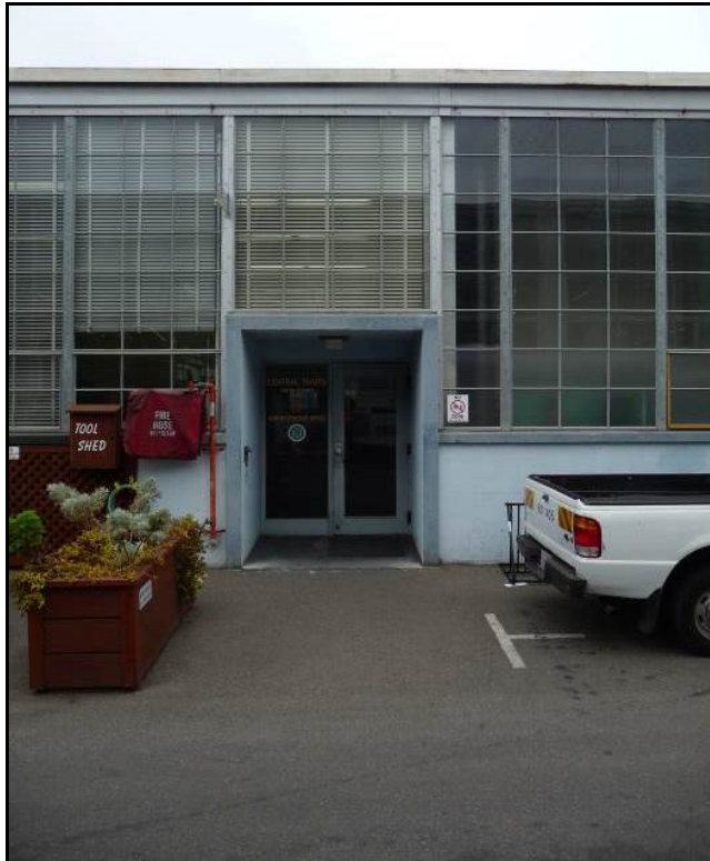
Photograph 4. Building A showing entrance to office area, camera facing southwest, August 20, 2014.
