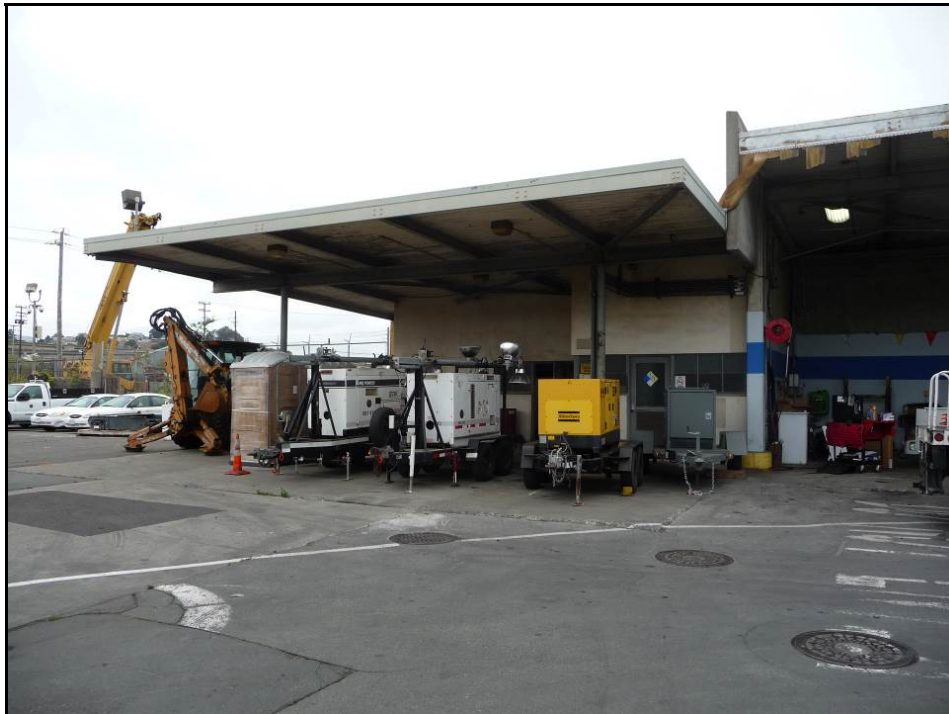
Photograph 11. Building C, north end, camera facing northwest, August 20, 2014.
