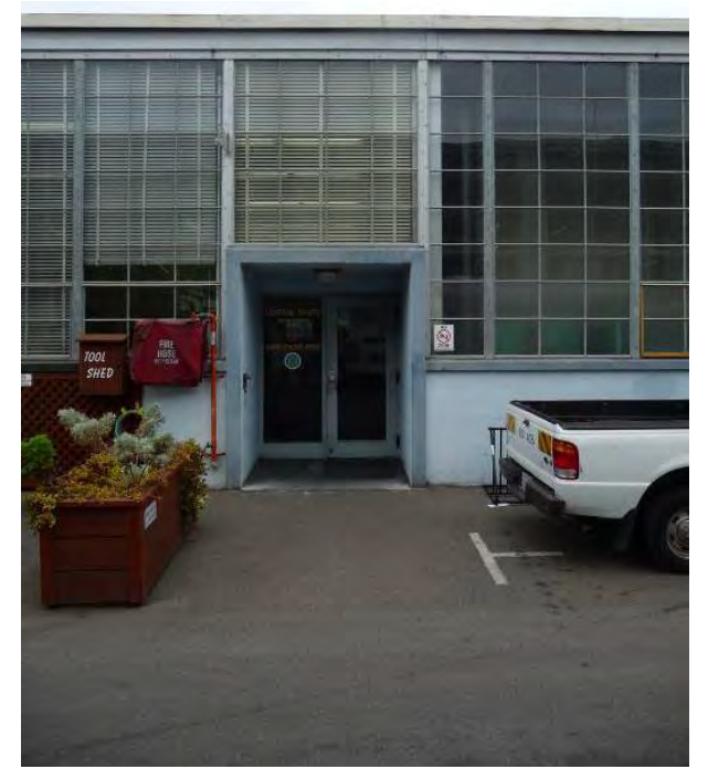
Building A facing southwest
