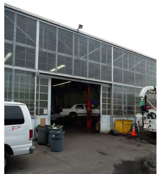
Building B facing northeast with car port
