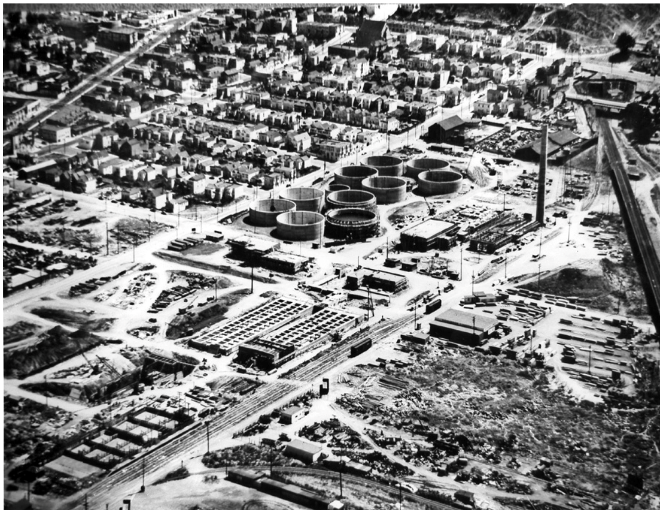
Figure 2. SEP Under Construction in 1950, Looking South.
