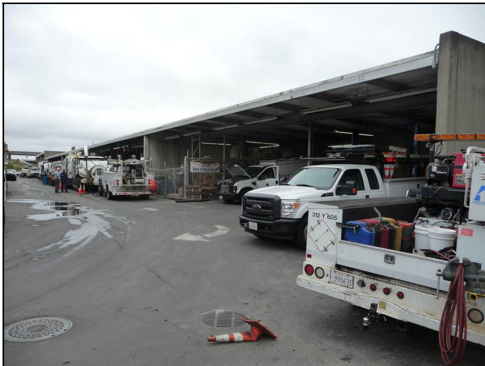
Photograph 9. Building C, camera facing northwest, August 20, 2014.
