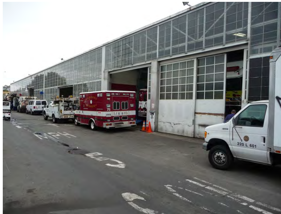
Building B facing southeast
