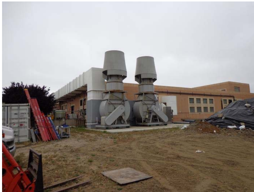
North and West Elevations (partial), Showing Newer Ventilation Shafts and Stacks
