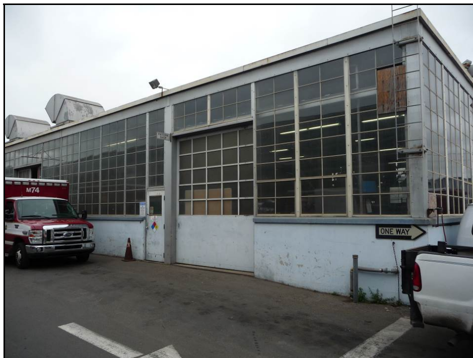
Photograph 3. Building A, north corner, camera facing southeast, August 20, 2014.
