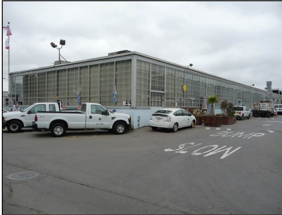
Photograph 2. Building A, camera facing west, August 20, 2014.
