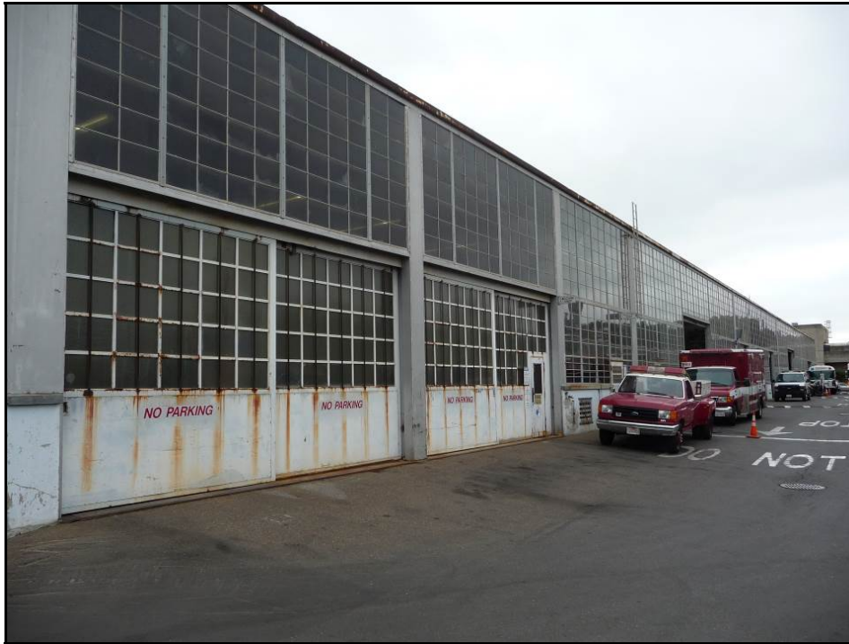
Photograph 6. Building B, camera facing northeast, August 20, 2014.
