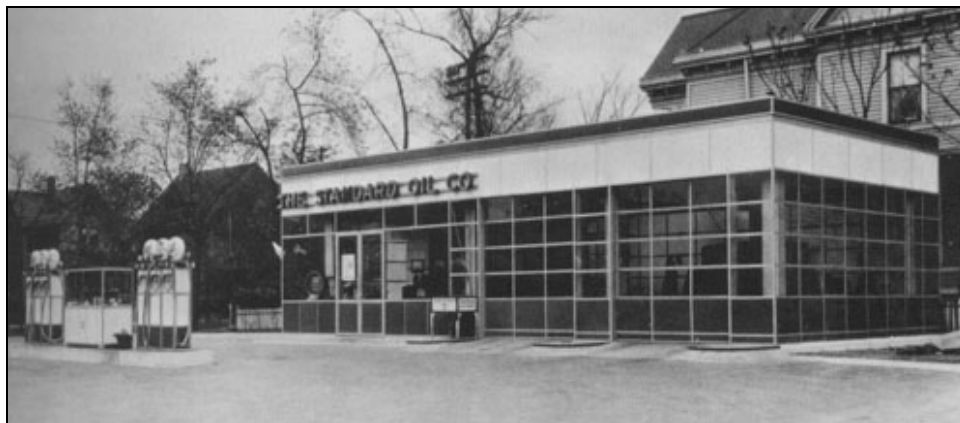
Figure 8: Filing Station, Standard Oil Company, Cleveland, Ohio, 1931. 28
