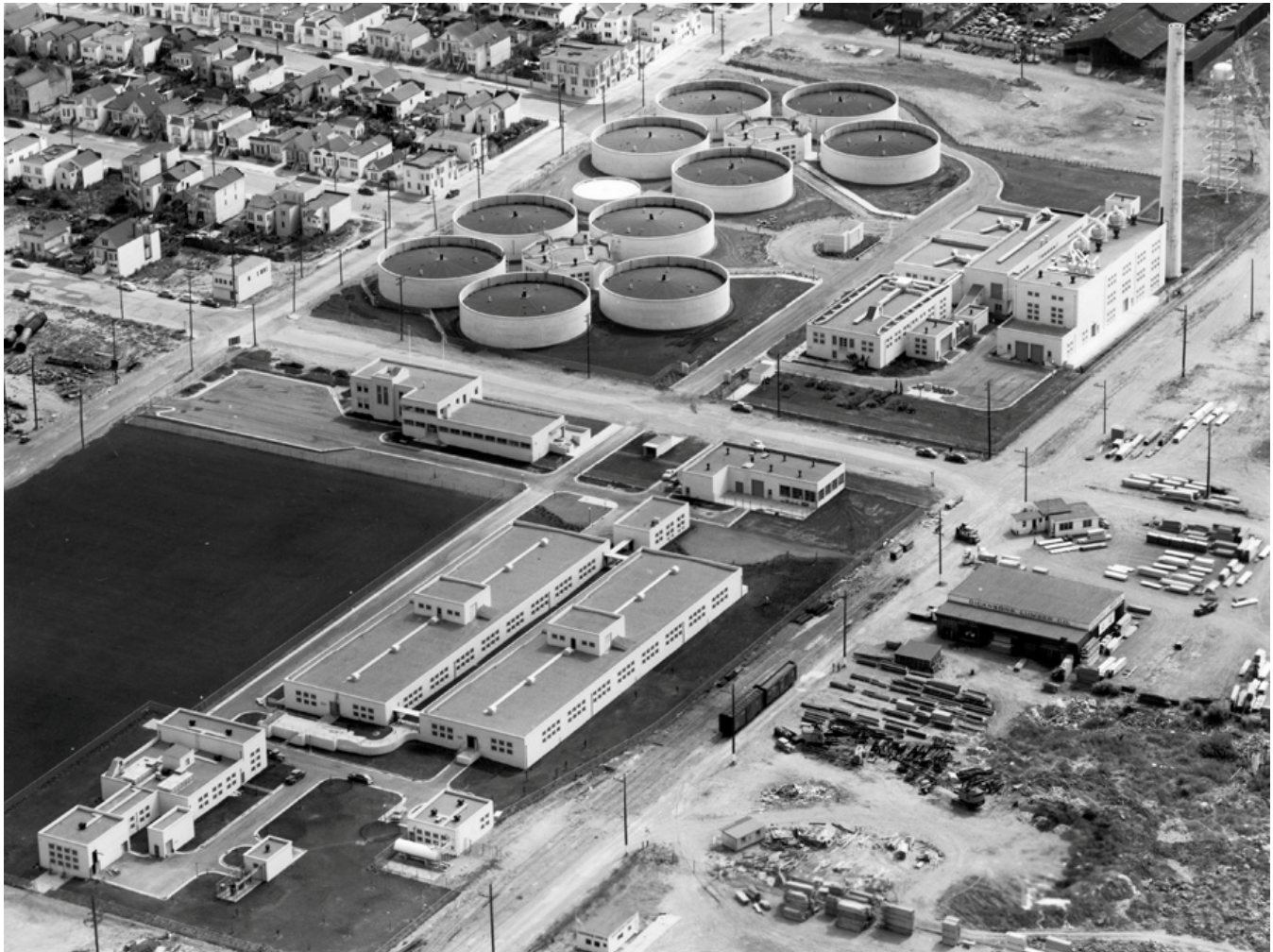
Figure 3. SEP Completed 1952, Looking South Source: SFPUC Photo Archives (Permission to Publish)
