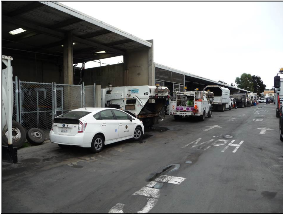
Photograph 10. Building C, camera facing east, August 20, 2014.
