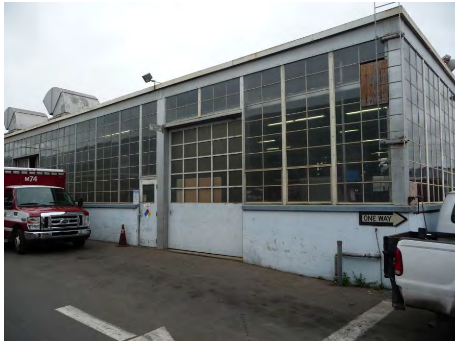
Building A facing southeast
